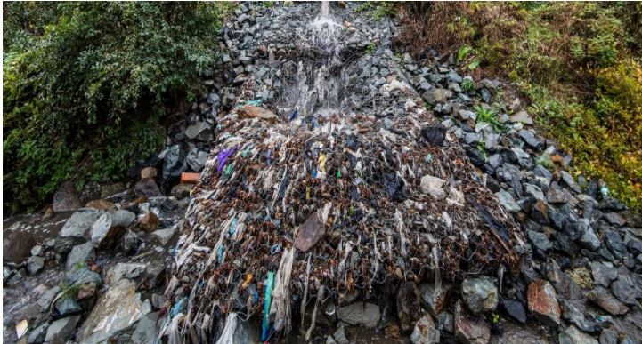
A sewage stream builds during a 10-hour spill outside Asheville, NC
