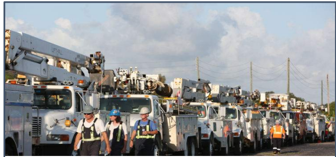
Power trucks head out from Derby Lane in St. Petersburg on Sept. 12, 2017, into Pinellas County to restore power after Hurricane Irma.
