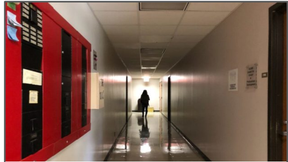
An emergency light inside a building at the University of Houston during a recent power outage.
