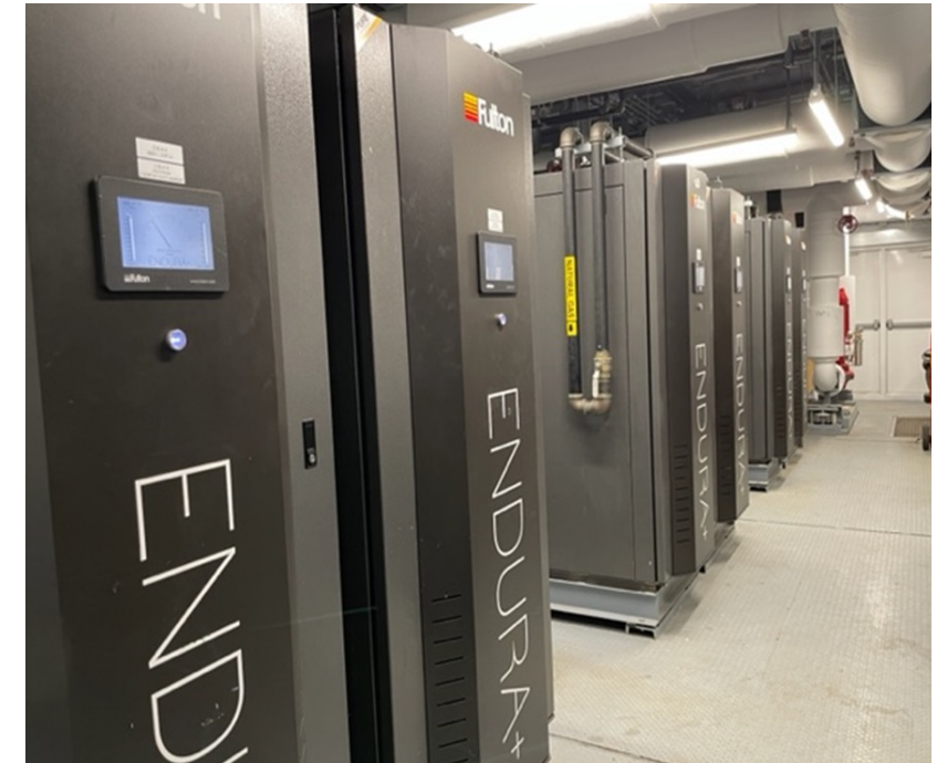
High Efficiency Condensing Boilers
