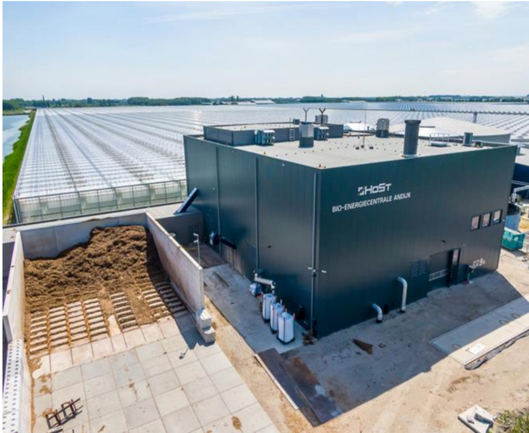
HoSt's 2020 State-of-Art Biomass CHP Plant: Produces 15 MW thermal + 3.4 MW electrical power
