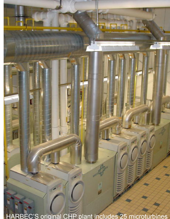
HARBEC'S original CHP plant includes 25 microturbines
